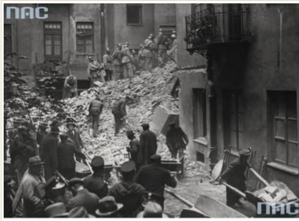
Rescue crews on the rubble of the Freta 16 annexe, August 1935. Photo: National Digital Archives.
