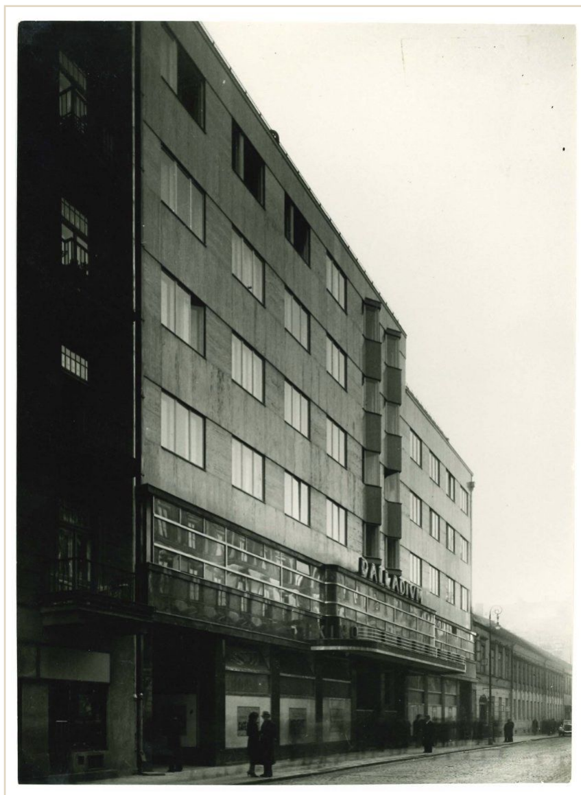
The building of Assicurazioni Generali Trieste, Złota 7/9, with the „Palladium” cinema — completed in 1937; the cinema's neon was hung the same year. The Zegrze family lived in it from the beginning.
