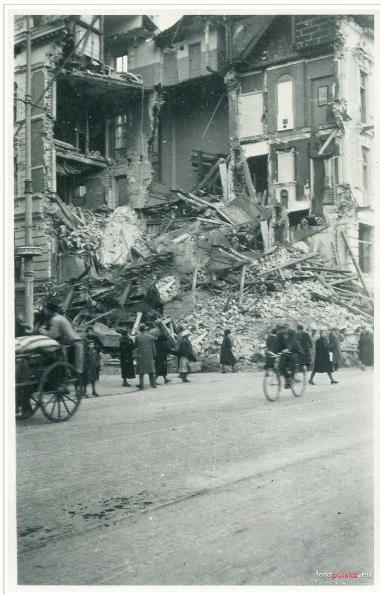
The street already passable: a cart, a cyclist, passers-by and children beneath the heap of beams and bricks that still lies on the pavement before the corner. The turn of 1939 and 1940. fotopolska.eu.
