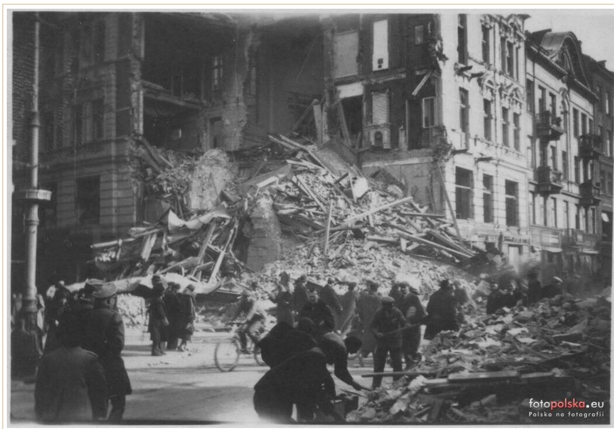
Clearing the rubble on Nowy Świat, autumn 1939: residents pick bricks and boards from the heap before the corner of no. 30; a cyclist rides past. fotopolska.eu.
